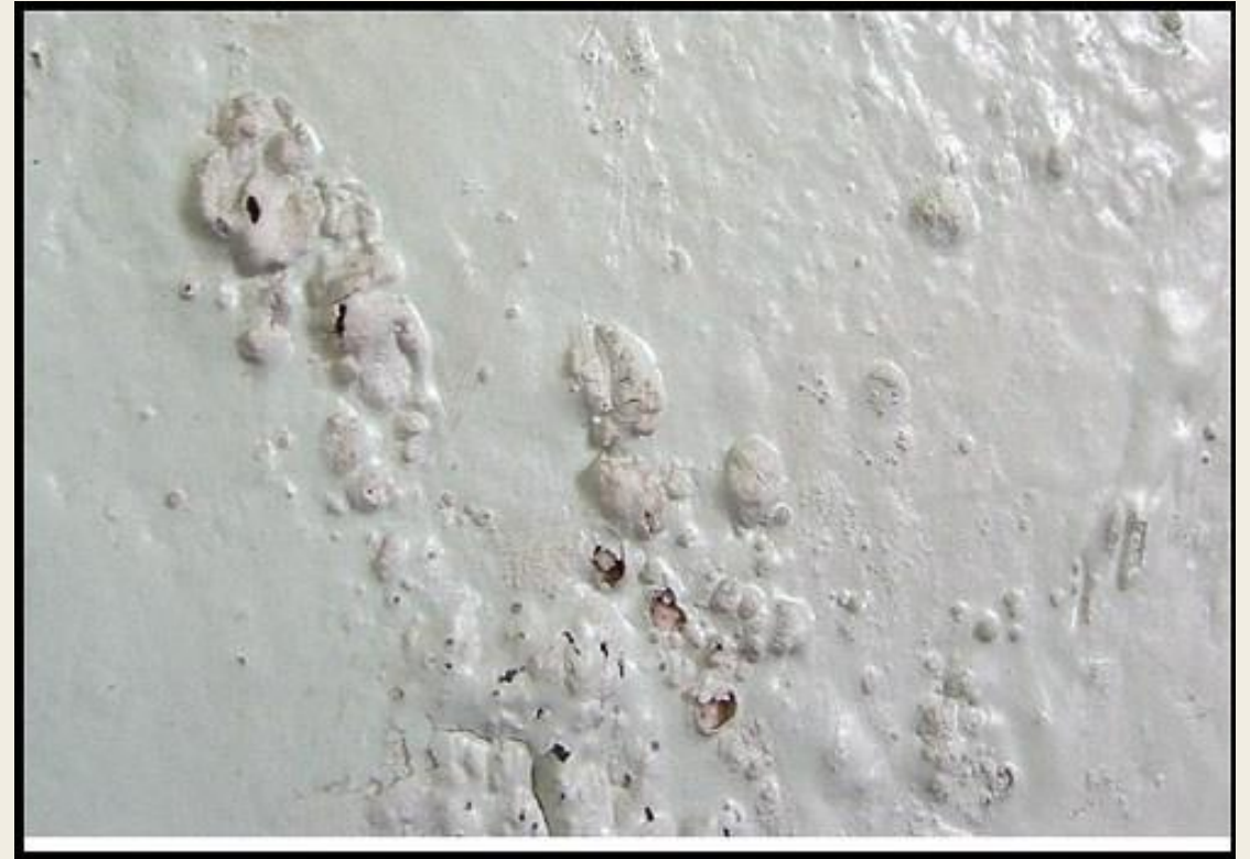
Efflorescence on a plaster wall
